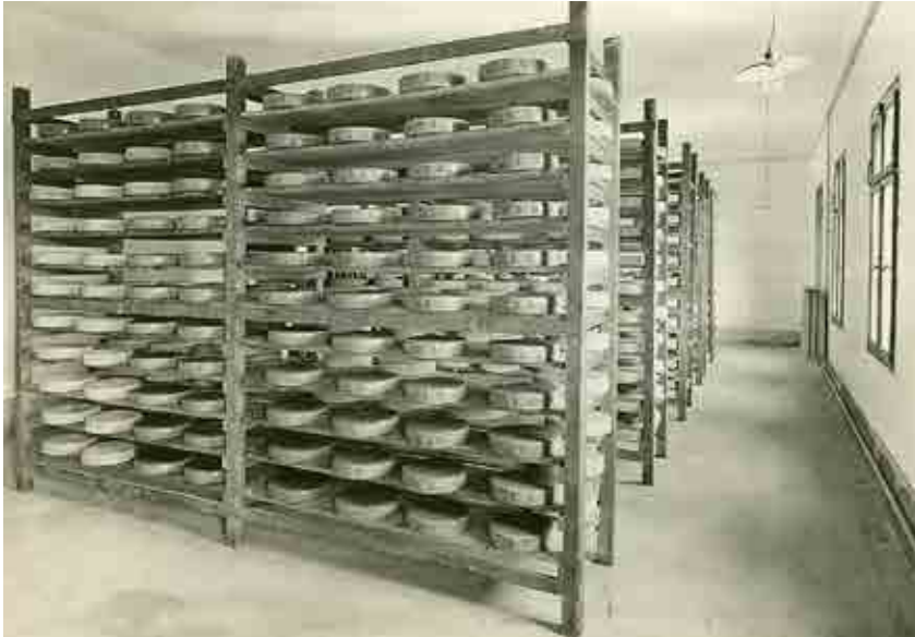
The warehouse of Vivaro dairy in the 1930s.
